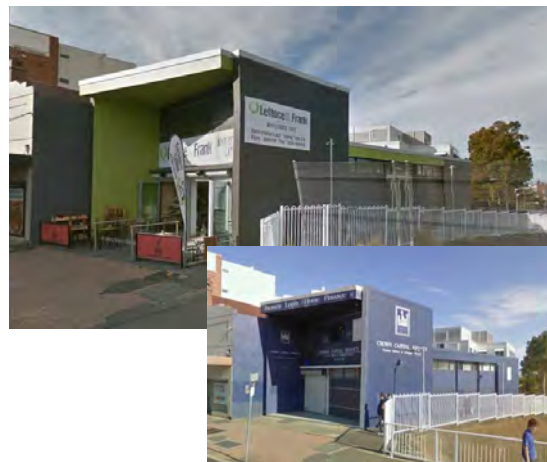
Fig. 3 Commercial building before (above) and after (below) upgrading.
