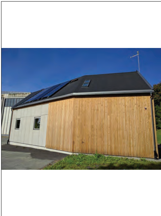
Fig. 1. The ZEB Test Cells Laboratory external view
