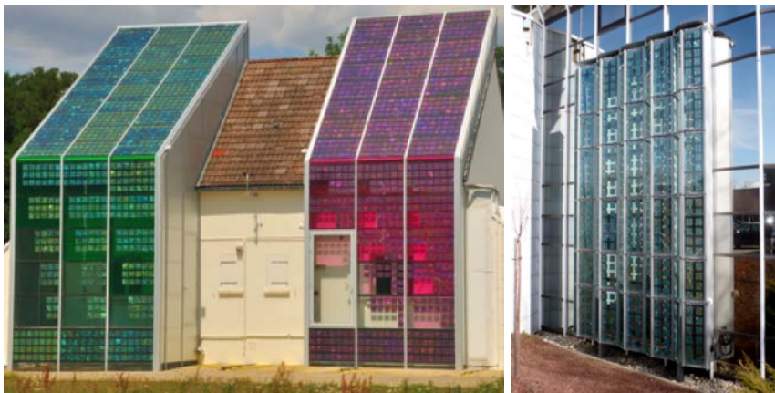
Figure 3. Double-skin prototype for detached houses (ETNA Test house – EDF R&D) - Pleated façade prototype for office buildings (HBS-Technal)
