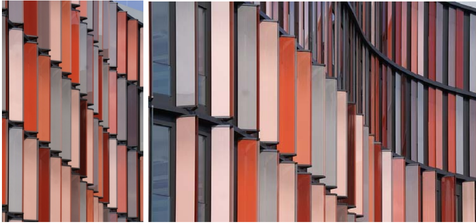
Figure 2. The Oval Offices in Cologne (arch. Sauerbruch and Hutton, 2010) The vertical axis glazed sun louvers serve the purpose of light regulation and, simultaneously, perform as outstanding architectural façade element. (photo by M. Brzezicki)
