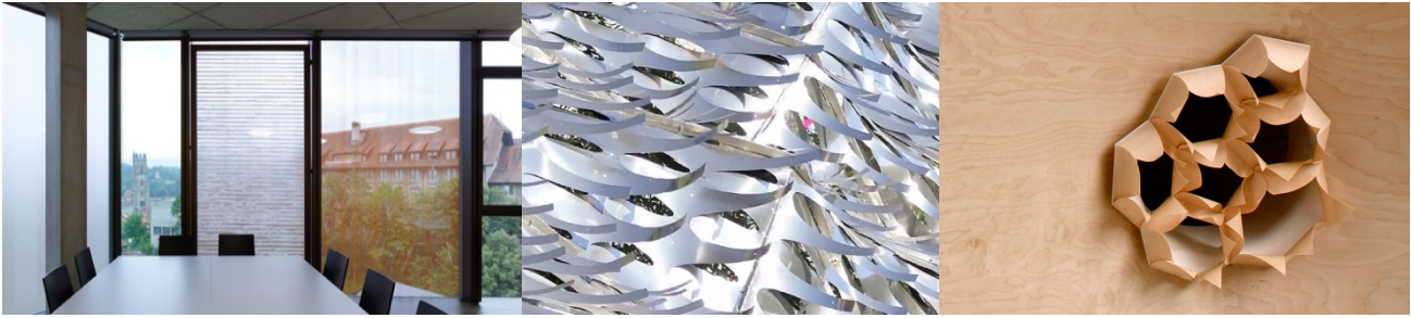
Figure 2: Various examples for self-responsive, smart materials in facades (from left to right): Centre Professionnel, Fribourg, CH, thermos-adaptive glazing by GlassX (phase change insulation, embedded in glazing system, that reacts autonomous on thermal changes) (Source: [4]); Installation “Bloom”, Los Angeles, USA, by Doris Kim Sung (laminated metal sheets with a thermo-bimetal behaviour that is activated by temperature differences) (Source: [5]); HygroSkin, permanent collection, FRAC Centre Orléans, FR, by ICD Uni Stuttgart (maple veneer composites that are shape-adaptive according to moisture content in air) (Source: [8]).
